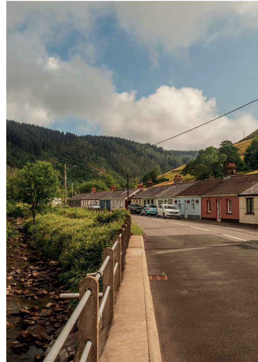
| Gelli Houses, Cymmer (Grade II Listed Buildings).
