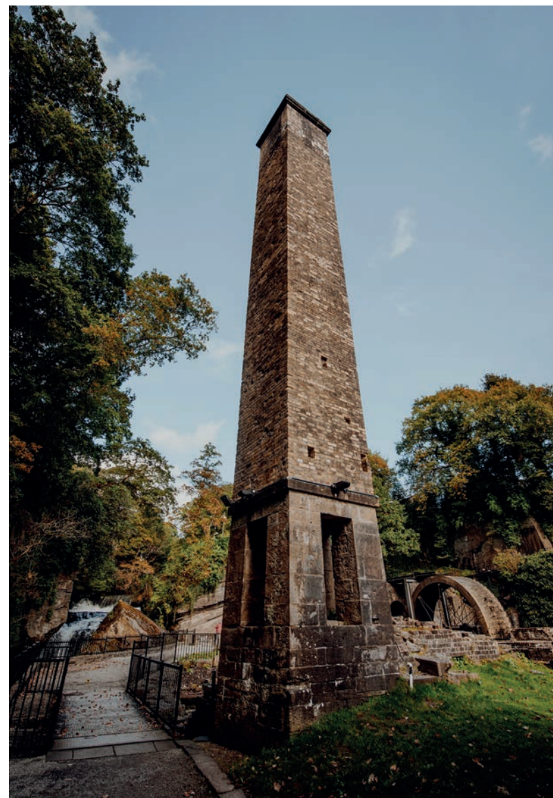
Chimney at Aberdulais Falls Tinplate Works (Grade II Listed Building).
